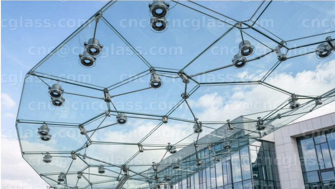
Figure 5 — Application: structural facade / canopy with irregular panels and point-fixed cutouts.
